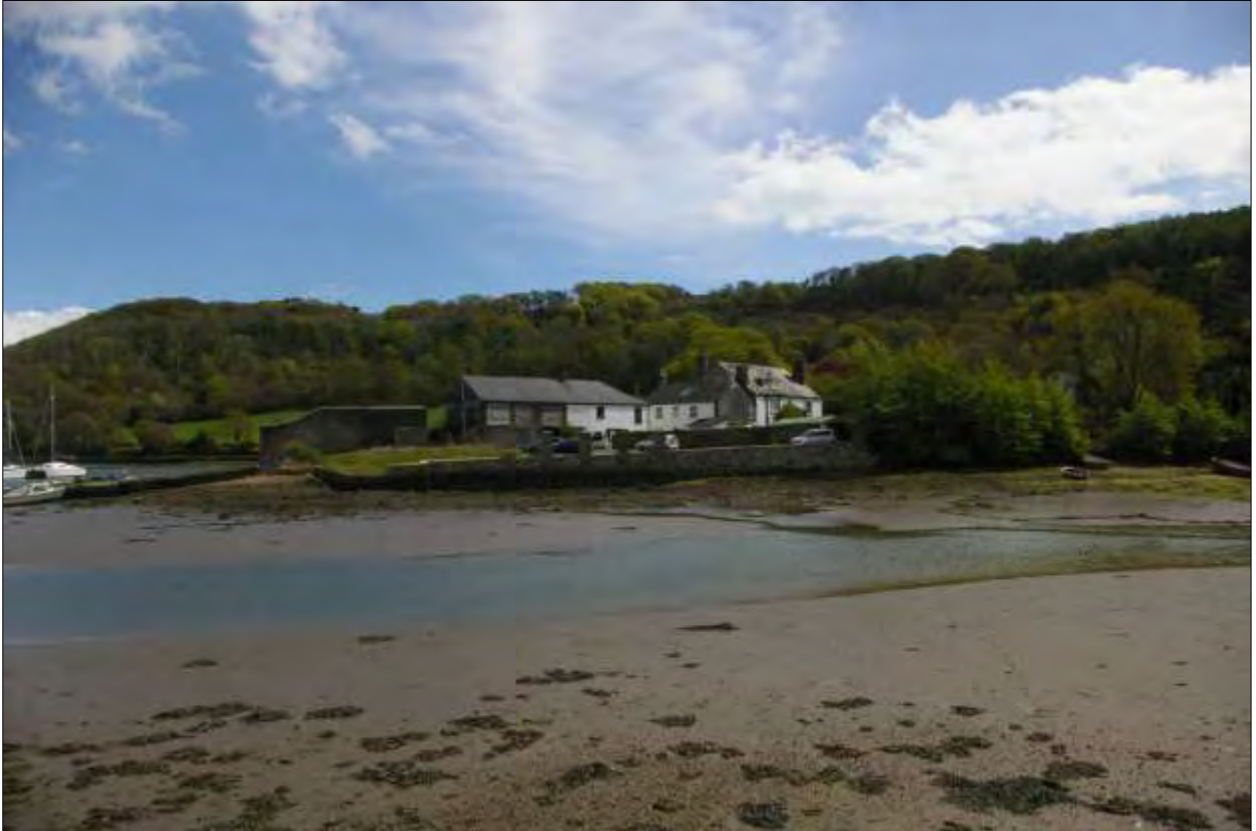
View of Anderton House; from the west, north-west.
