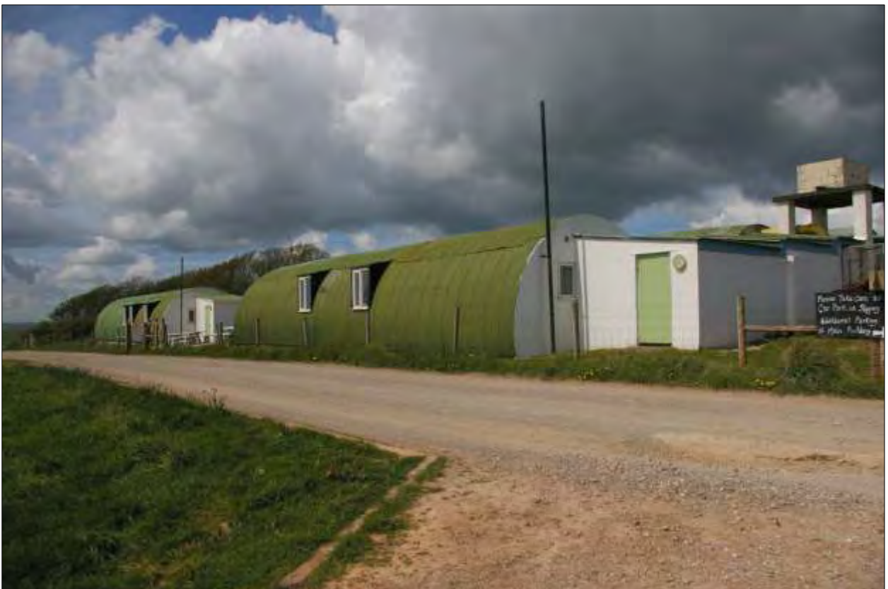
The second of the batteries, now with WWII buildings on it, at Maker Heights; from the south.
