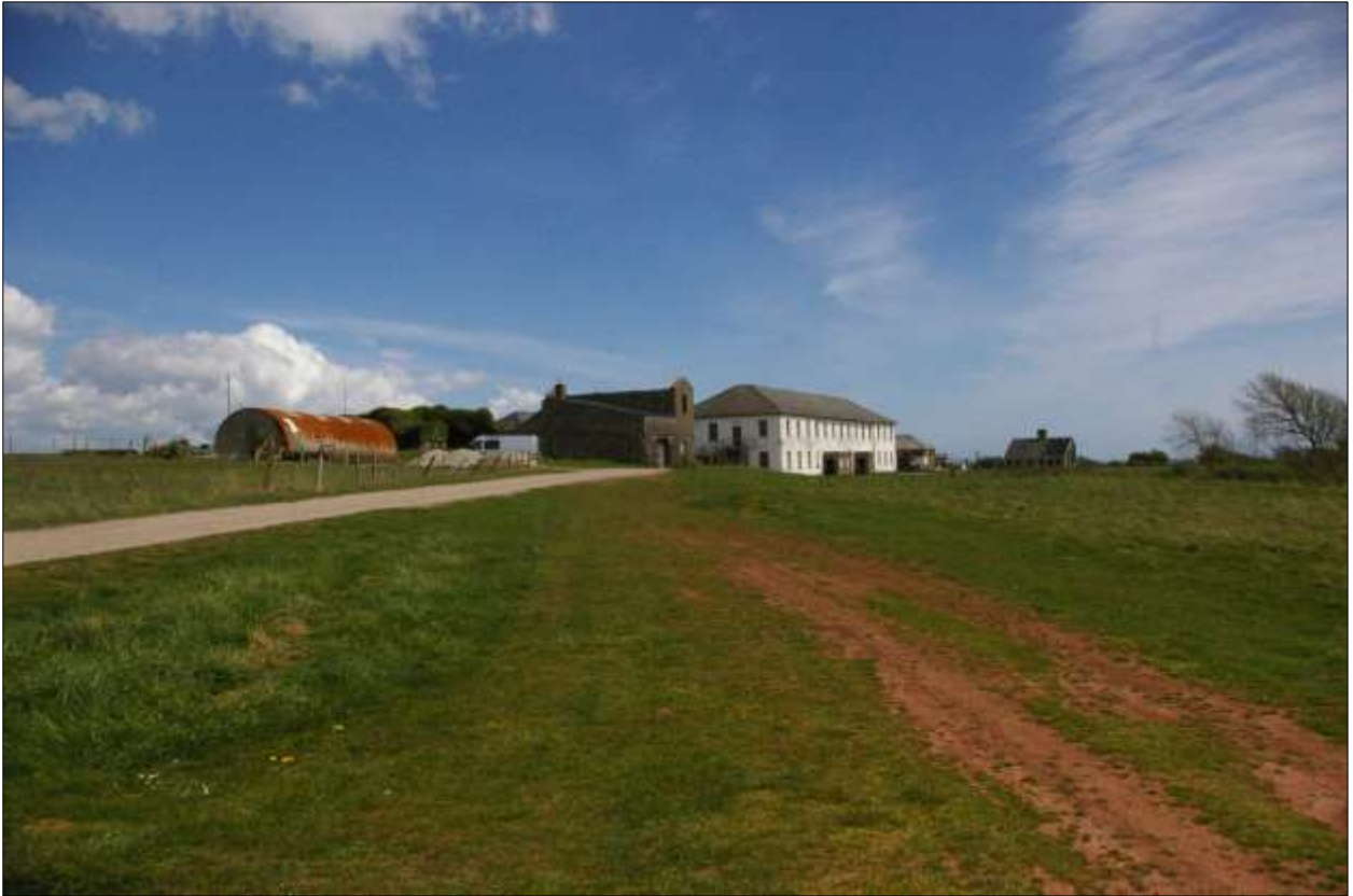
One of the batteries at Maker Heights, with the Grade II* Listed buildings; from the north-west.
