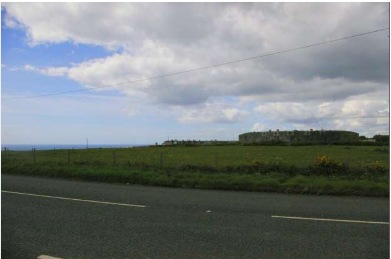
Tregantle Fort, on the high ridge, looking out to sea; from the east.
