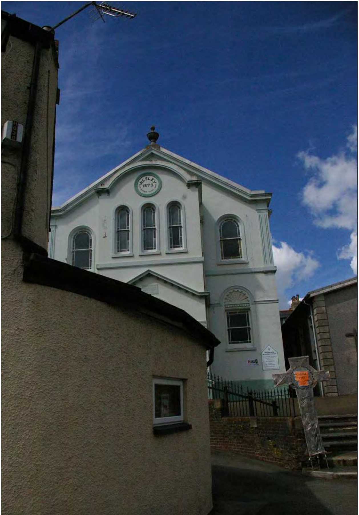
The south front of the Methodist Church; from the south.
