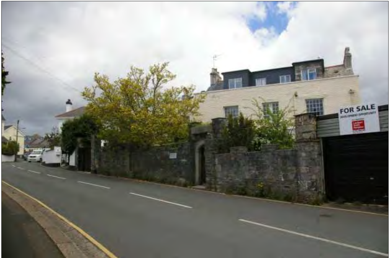
Grade I Listed archway within wall along Culver Road in Saltash; from the south-east
