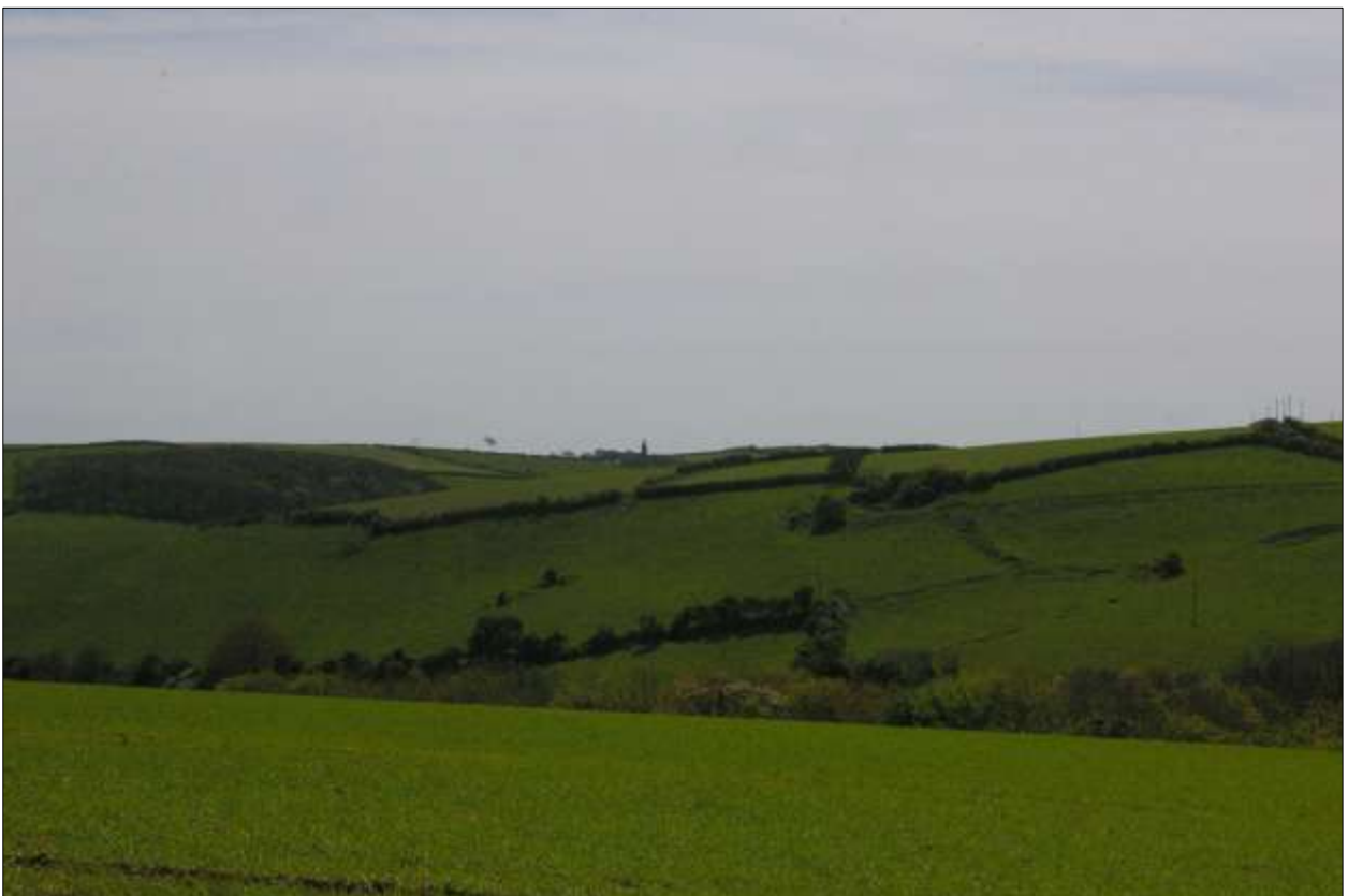
The tower of St. Germanus, Rame; emphasising its complete landscape dominance on the headland of the peninsula; from the east.
