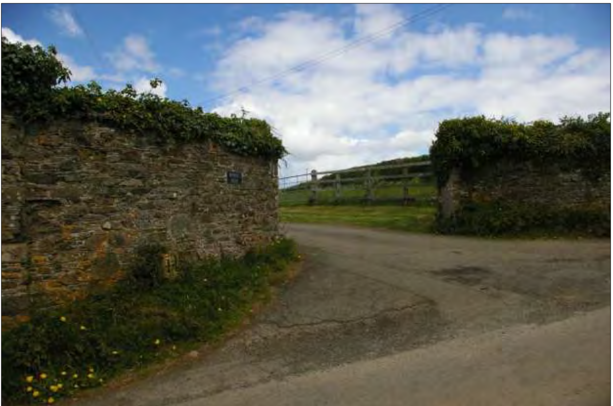
The stone wall and gate piers which frame the long drive to Burrell House; from the south-west.
