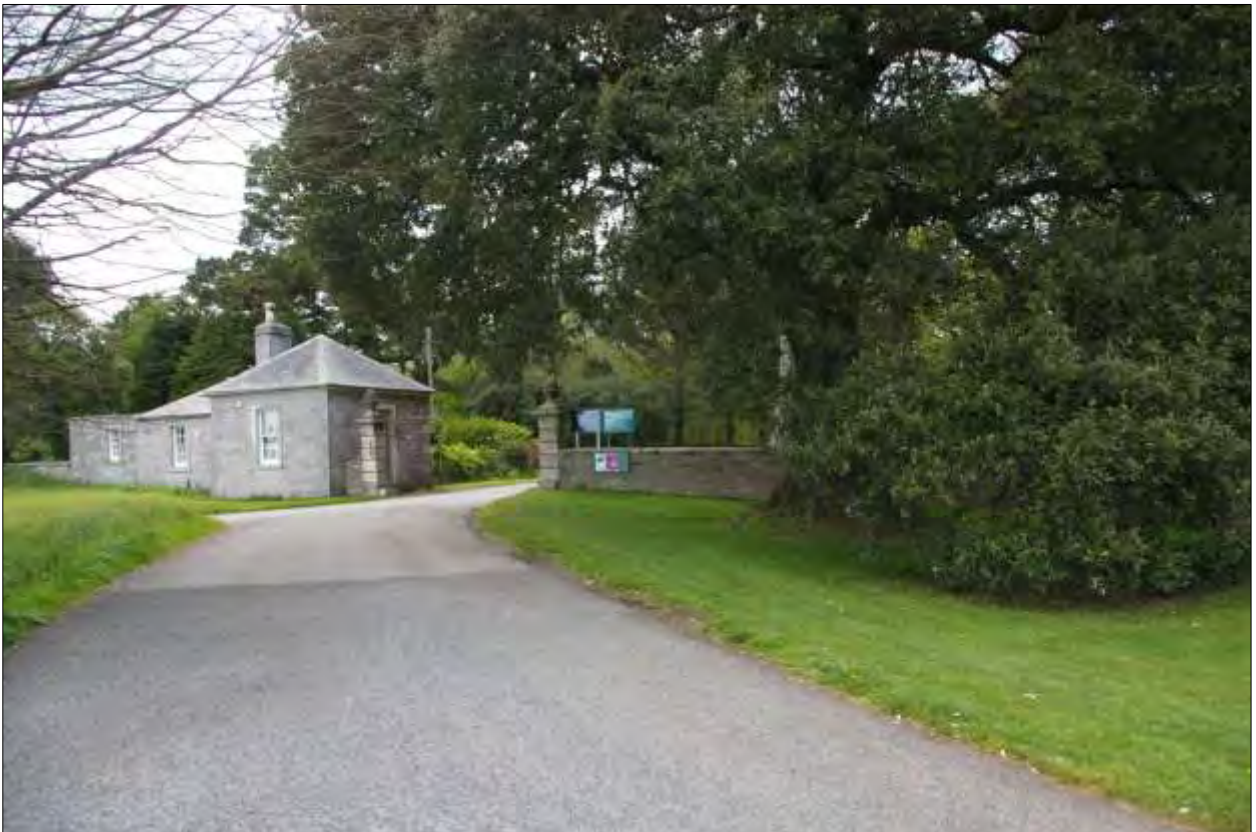
View of the main entrance to the Antony Estate; from the south-east.
