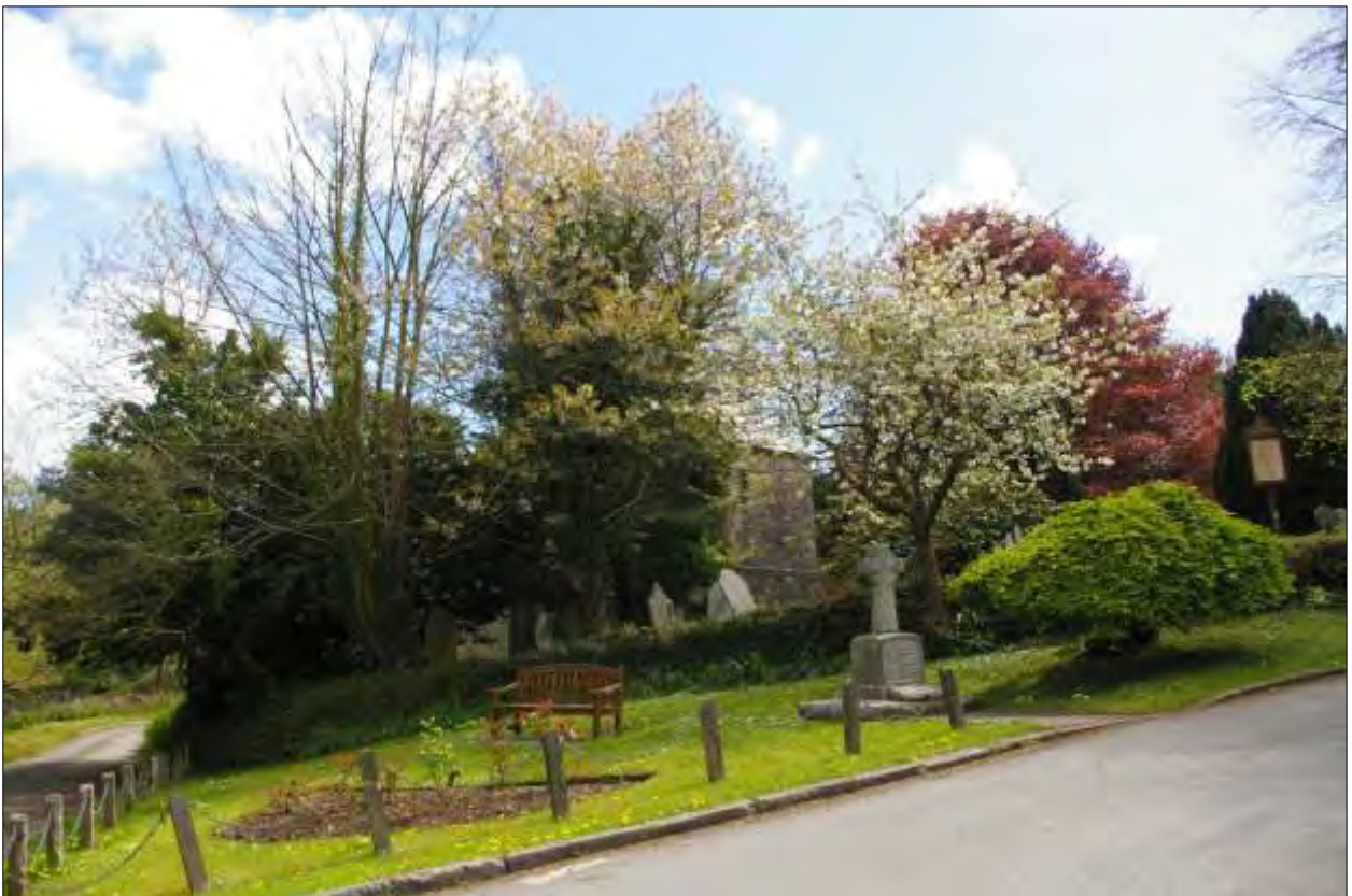
View of the church of St John, in the heart of the Conservation Area, located in the base of the valley; from the north-west.
