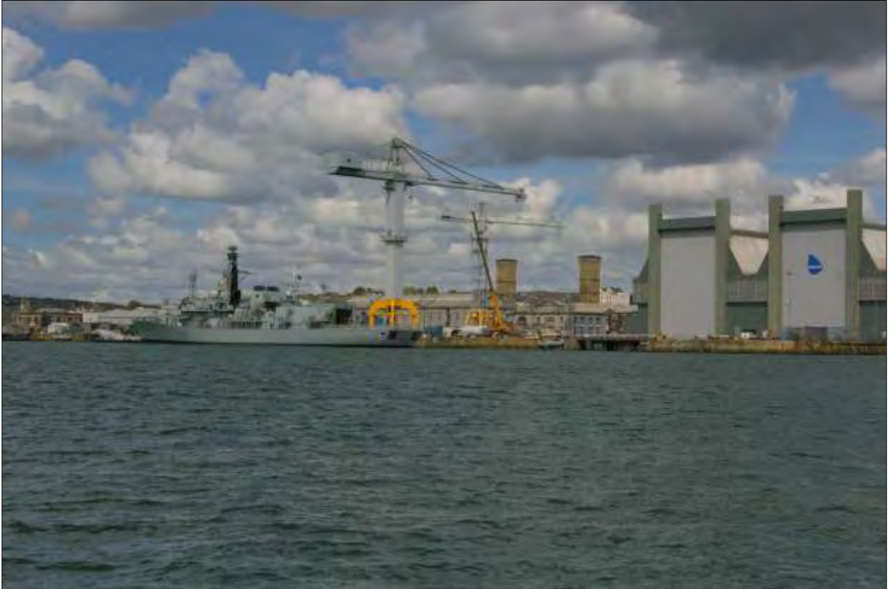
View of the long frontage of the Quadrangle, amongst the modern impacts of the Devonport Docks; from the south-west.
